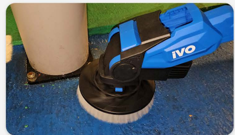
Industrial Flooring Detail
